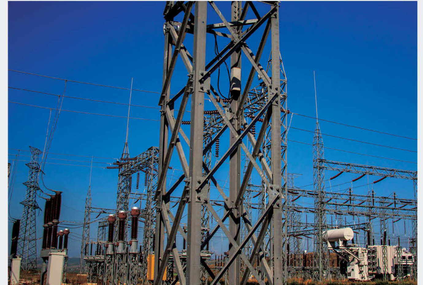
The expansion of Babice Substation
