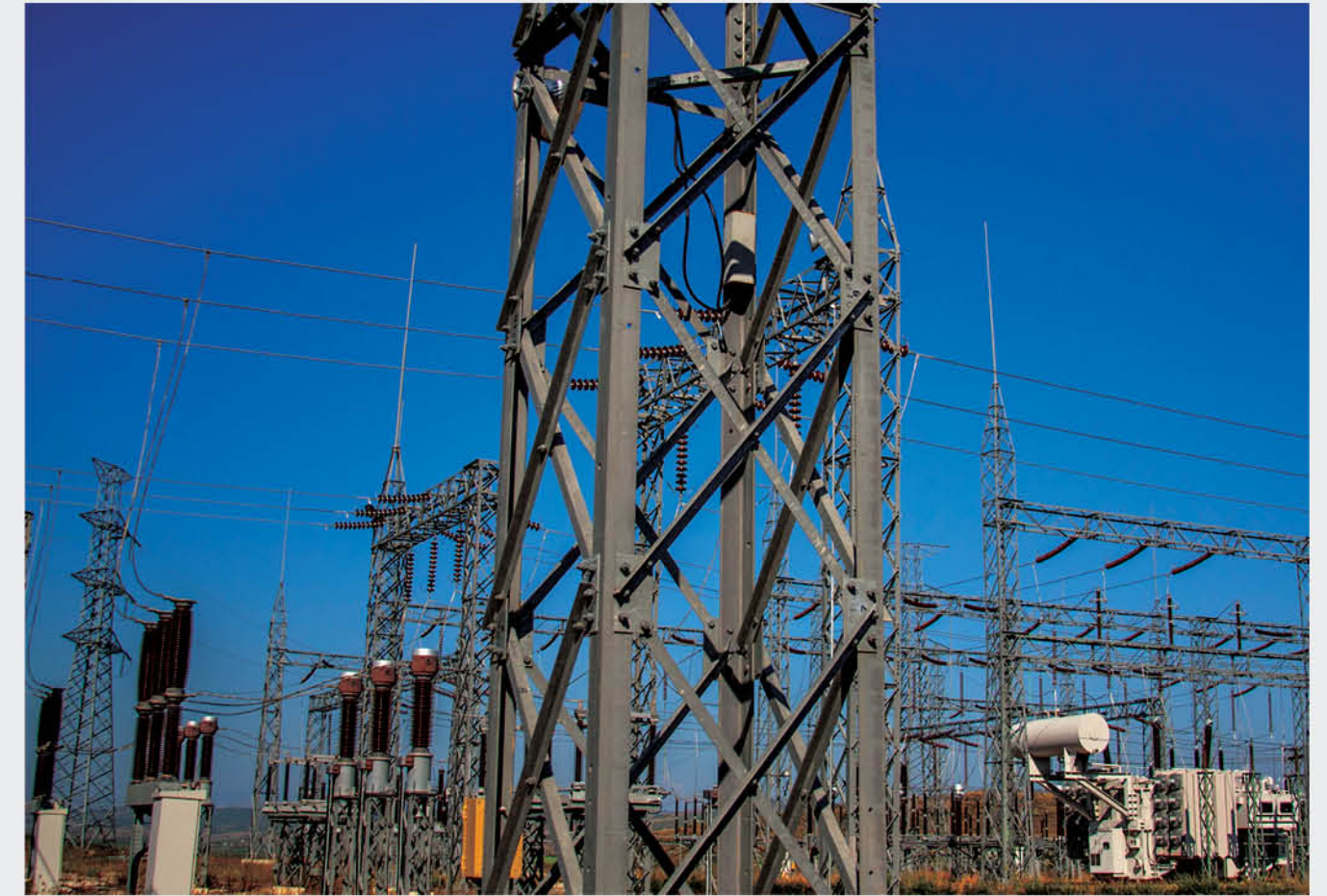
The expansion of Babice Substation
