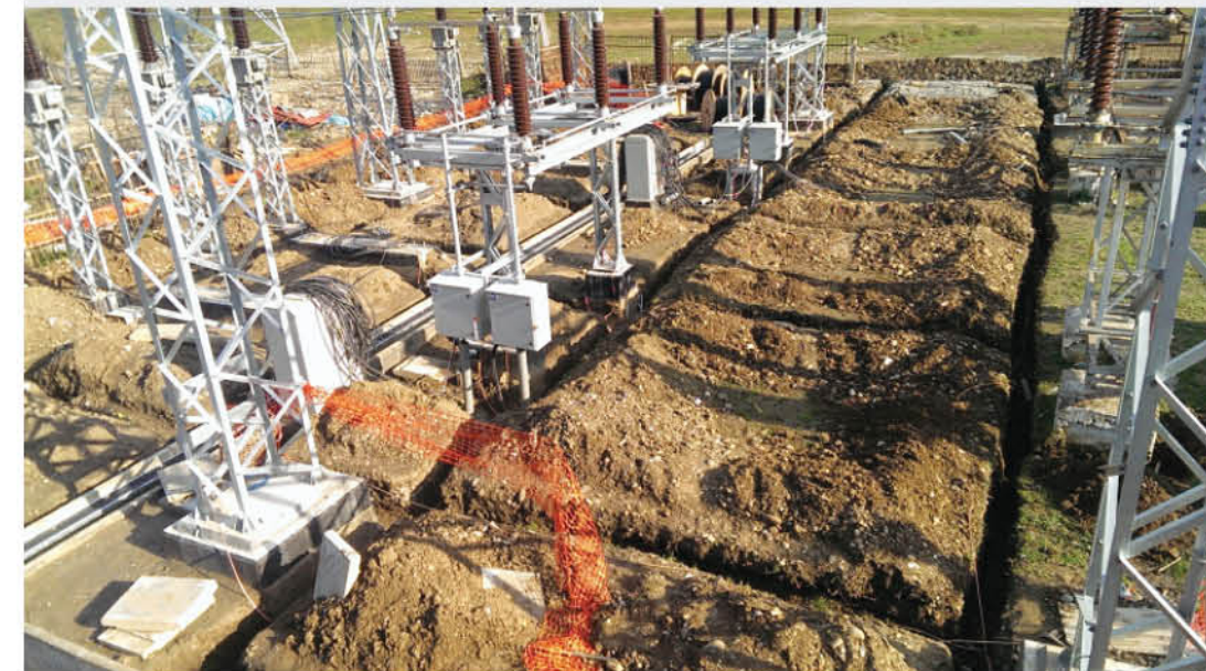
Earth system in Permet substation
