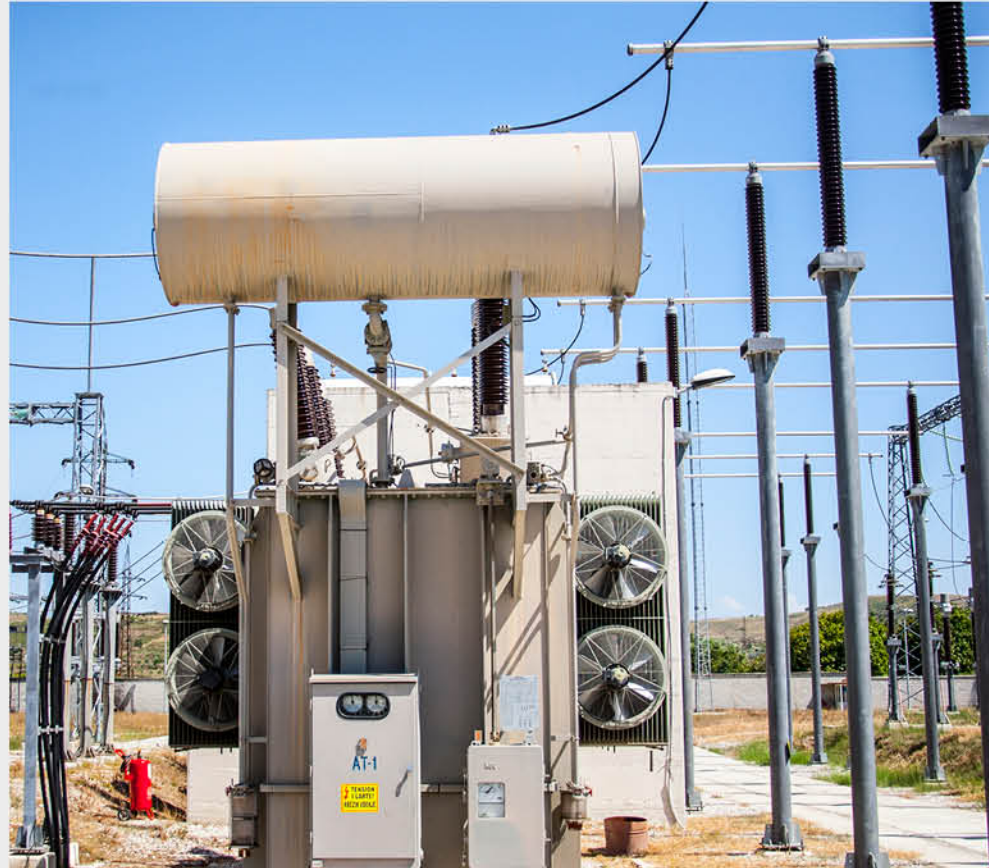
The installation of the new 150 MV transformer in Zemblak substation
